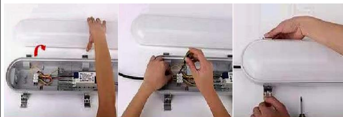
1)Open the Cover/Diffser 2)Connect the Wire 3)Close the Cover/Diffser
